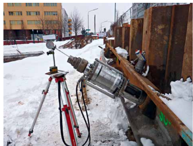
12 Example of the anchor installation during tensioning by an hydraulic jack and strain measurement (Source: Porr Bau GmbH)
