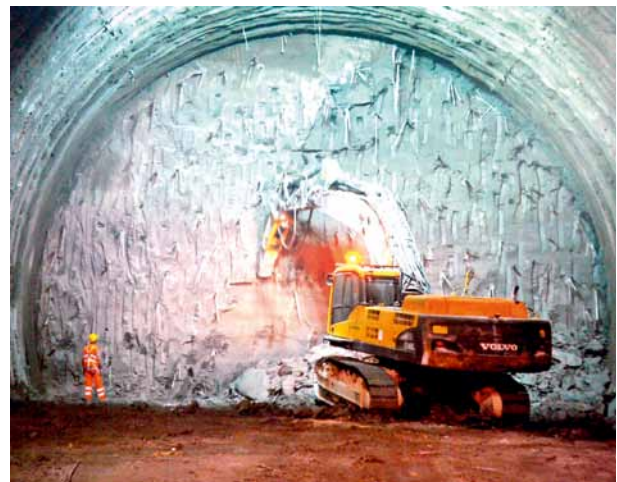
6 Tunnel face during excavation
