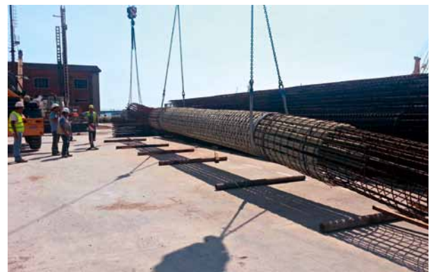
9 Napoli Port – GFRP pile cage during lifting operations (Source: Società Italiana per Condotte d'Acqua S.p.A.)
