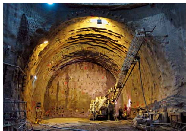
15 Tunnel face with drilling machine during the first excavation and installation of GFRP flat-bars anchors. A portion of the vertical shaft border is visible in the upper part (Source: Consolidations Suisse)
